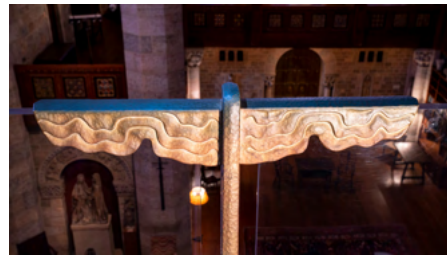
Monel balcony railing
