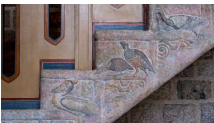
Poured concrete stairs
